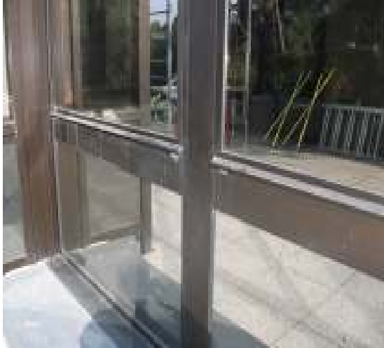
Before treatment the anodized finish has lost its lustre
